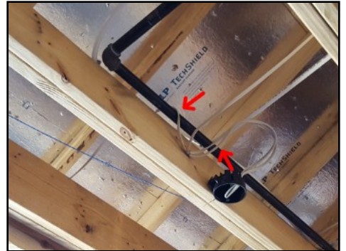
Protect wire from gas line at master closet
