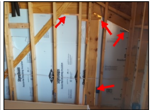
Gaps in thermal barrier/Not secure
