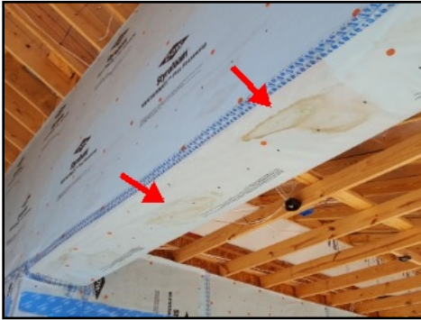
Moisture trapped within vapor barrier/Stains present
