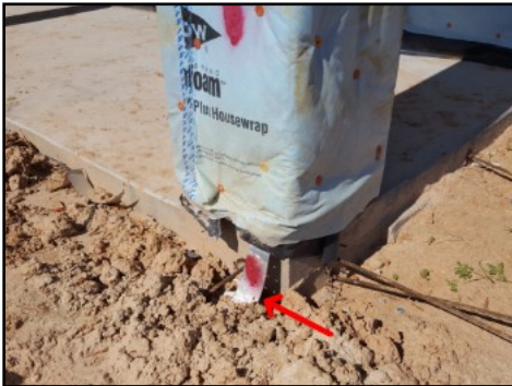
Windstorm brace not secure at rear left elevation
