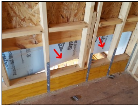
Thermal barrier not secure in place
