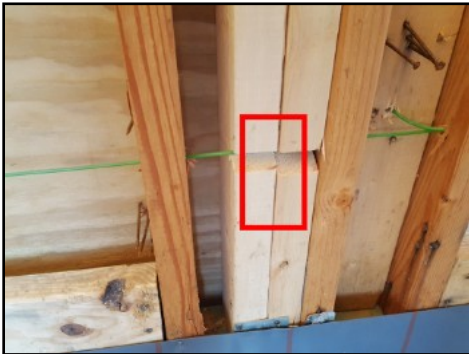
Missing metal tie/strap at master bathroom shower
