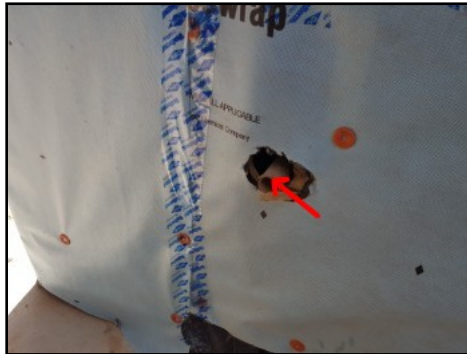
Seal all exterior penetrations
