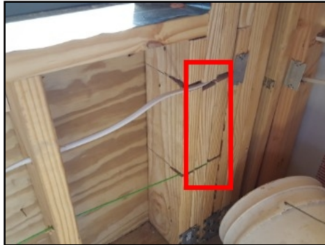
Missing metal tie/strap at living room
