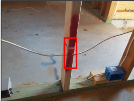
Missing metal tie/strap at lower media room
