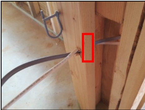
Missing nail guard at master bedroom hallway
