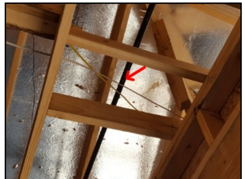
Protect wire from gas line at garage
