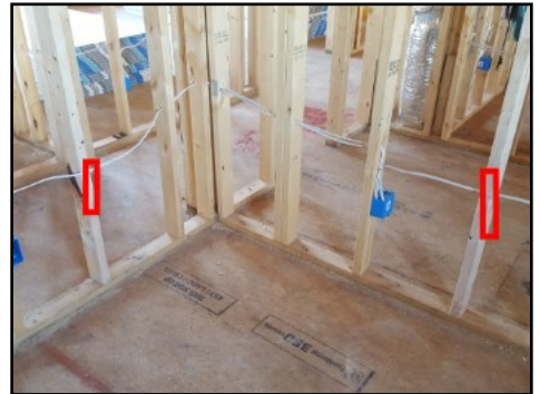
Missing metal tie/straps at upstairs hallway closet
