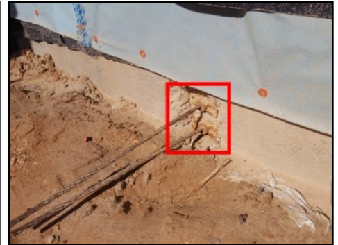
Exposed live end at rear elevation
