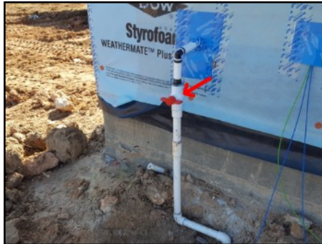
Main water shut off valve
