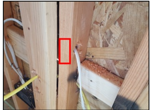
Missing nail guard at morning area
