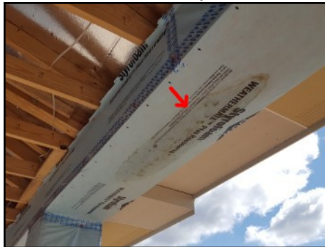
Moisture trapped within vapor barrier/Stains present
