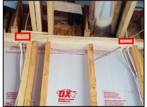
Missing nail guards at garage
