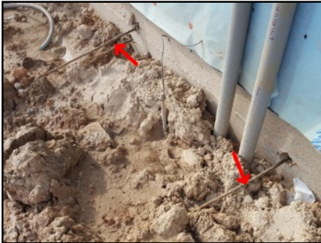
Cables not cut/sealed
