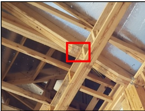
Notched rafter beam at front entry/dining room
