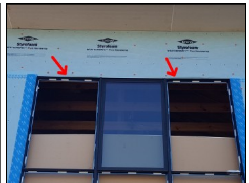
Upper jamb not flashed/taped
