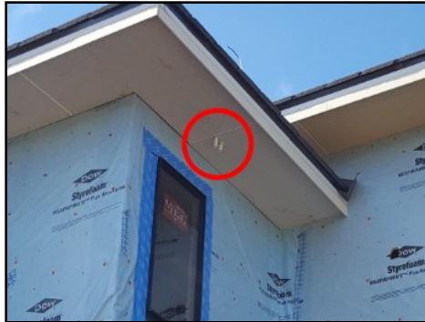
Secondary drain lines at front elevation
