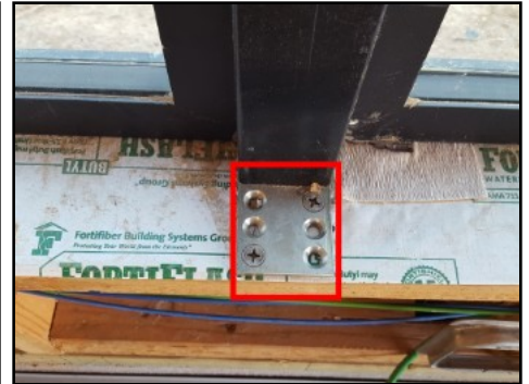
Missing securing hardware at window bracket
