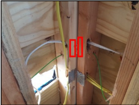
Missing nail guards at morning area
