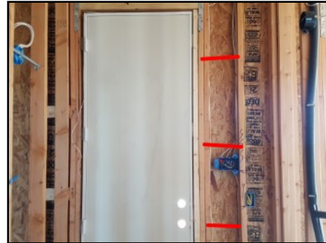
Recommend adding blocks on right side
