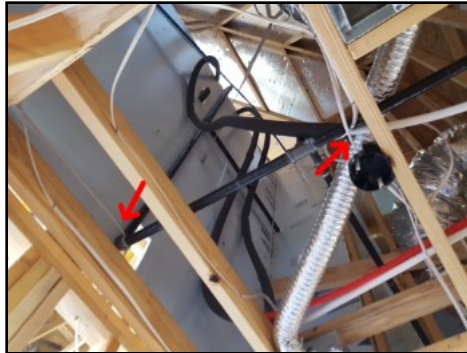
Protect wires from gas line at powder bathroom
