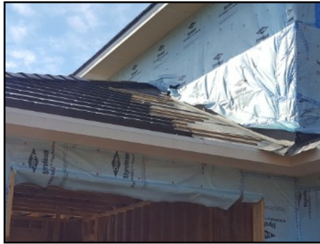
Roof covering not complete
