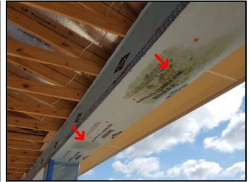
Moisture trapped within vapor barrier/Stains present
