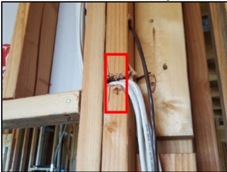
Missing nail guard at master bedroom
