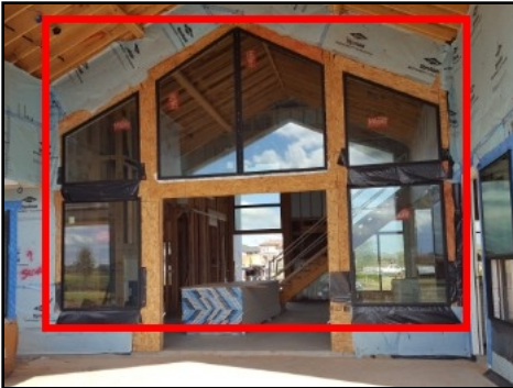
Window jambs not flashed/taped
