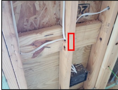
Missing nail guard at pool bathroom
