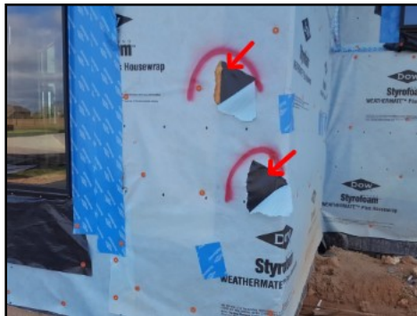
Repair/Seal vapor barrier at front elevation
