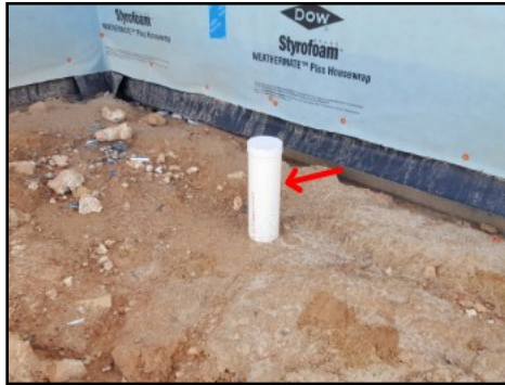
Main sewer clean at front right elevation
