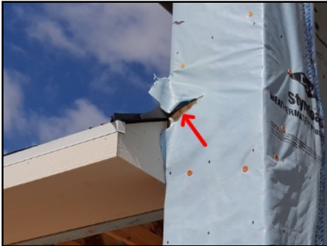
Secure/Seal vapor barrier at rear elevation
