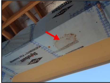
Moisture trapped within vapor barrier/Stains present
