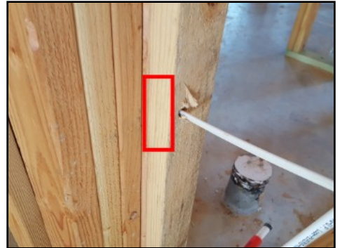
Missing nail guard at living room
