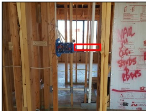
Junction box not blocked/secure
