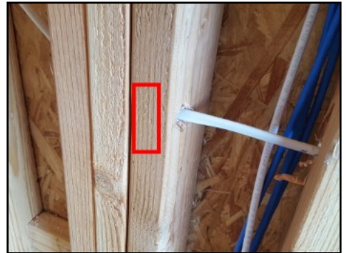
Missing nail guard at master bedroom
