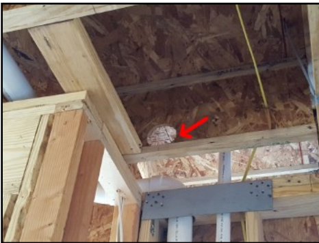
Boring to low at utility room joist
