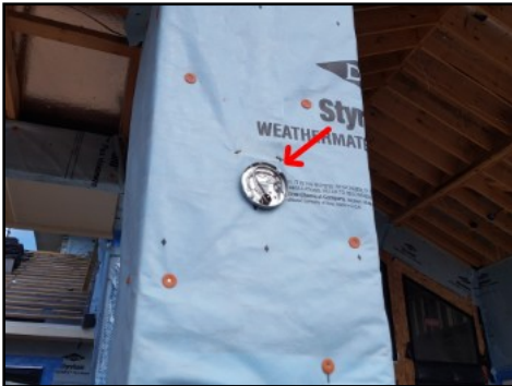
Seal all exterior penetrations
