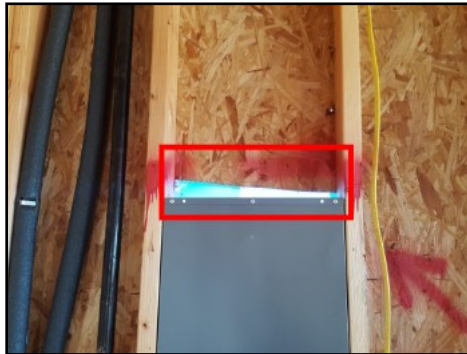
OSB not blocked in master closet
