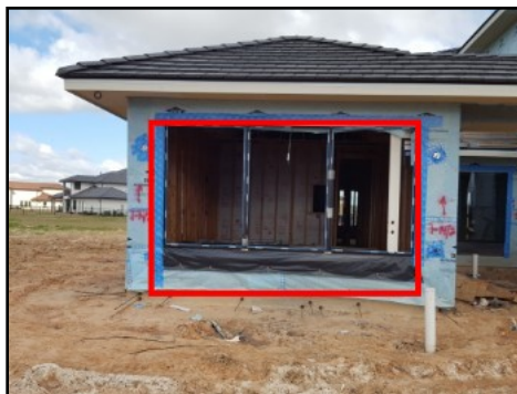
Glass not present at rear elevation
