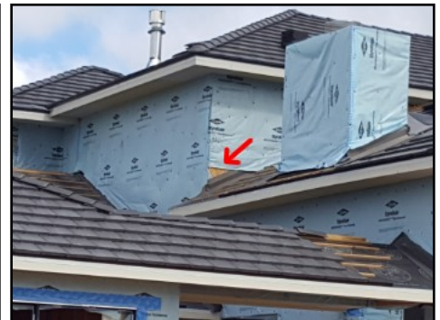
Repair/Seal vapor barrier at upper rear elevation
