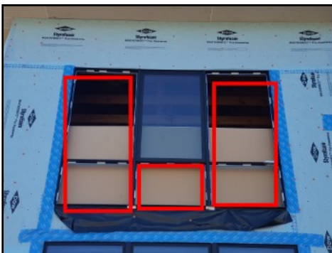
Glass not present at front elevation
