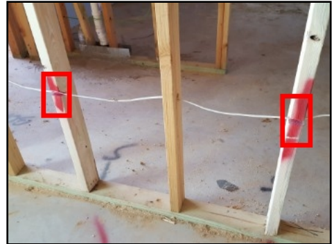
Missing metal tie/straps at study
