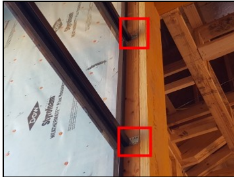
Missing securing hardware at window bracket
