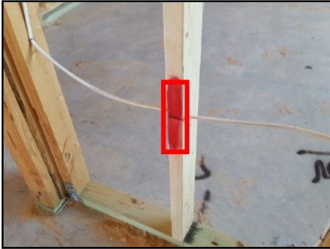
Missing metal tie/strap at lower level closet
