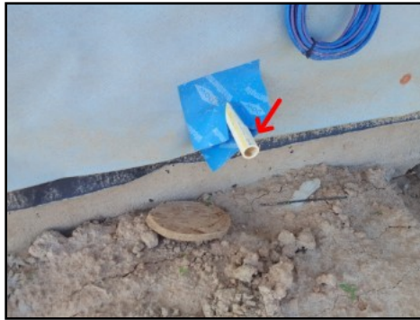
Drain line termination at left elevation
