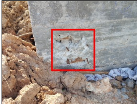
Exposed dead end at front left elevation
