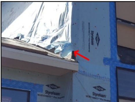
Secure/Seal vapor barrier at front left elevation
