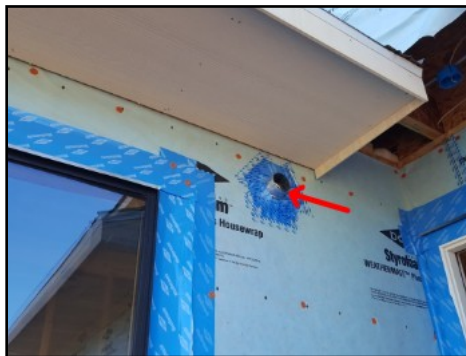
Dryer vent termination
