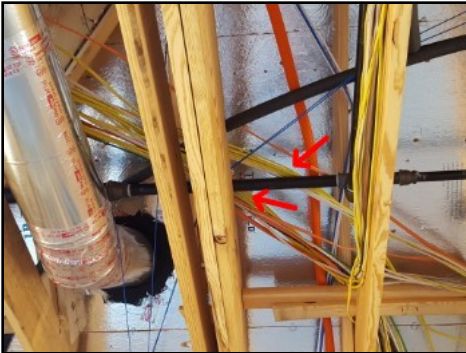
Protect wires from gas line at garage
