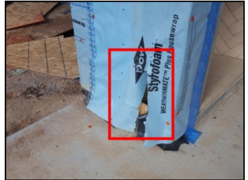
Repair/Seal vapor barrier at rear elevation
