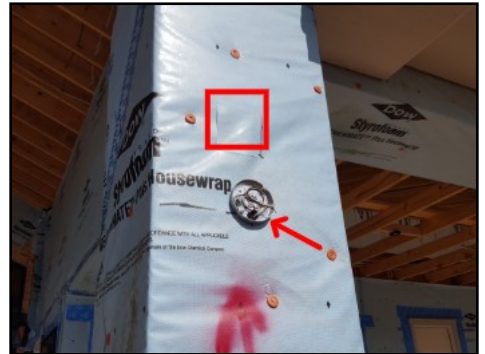
Seal all exterior penetrations/Repair
