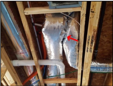
HVAC ducts in contact with one another
