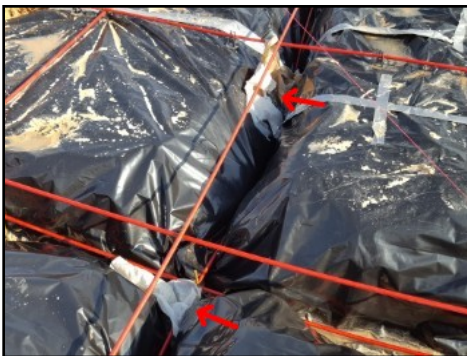
Remove all debris from within foundation
