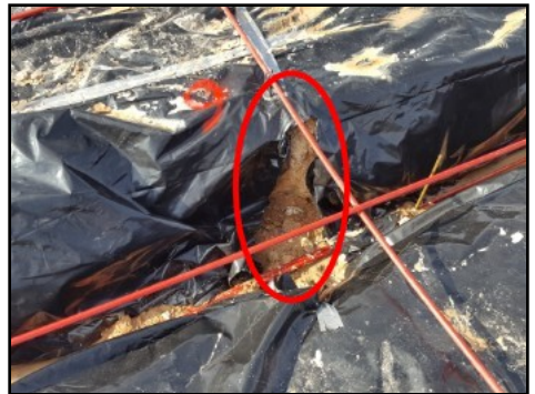
Repair/seal torn poly
