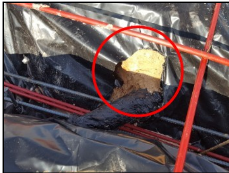
Repair/seal torn poly
