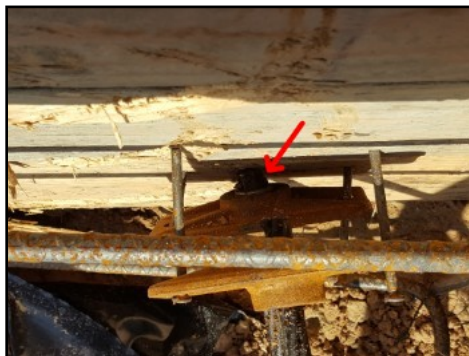
Cable in contact with form at left elevation
