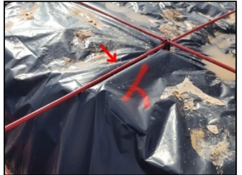
Cable not raised off pad
