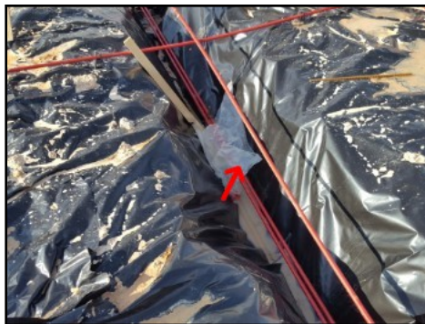
Remove all debris from within foundation
