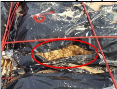
Repair/seal torn poly
