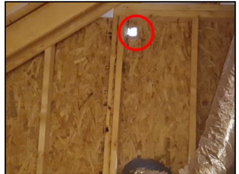
Seal hole at lower rear right attic space
