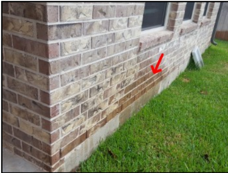
Sprinkler spraying structure
