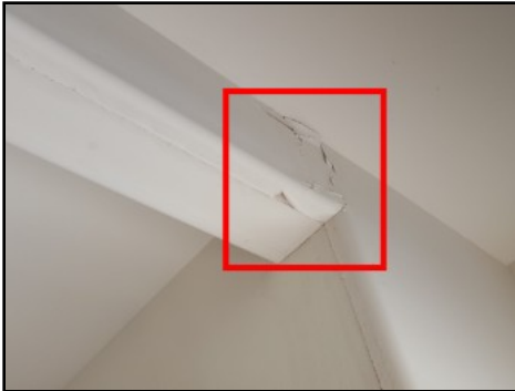
Moisture stains/damage present
