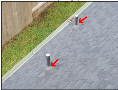
Buckled roof jacks at rear left elevation
