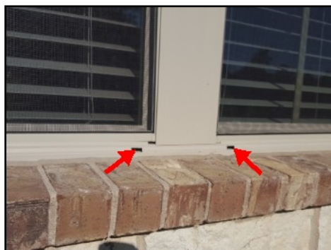
Missing weep hole covers at front elevation
