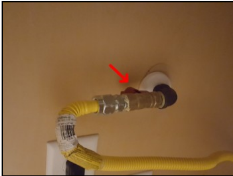
Gas line service valve is beneath unit
