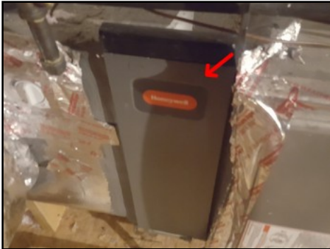
HVAC media filter location/hatch
