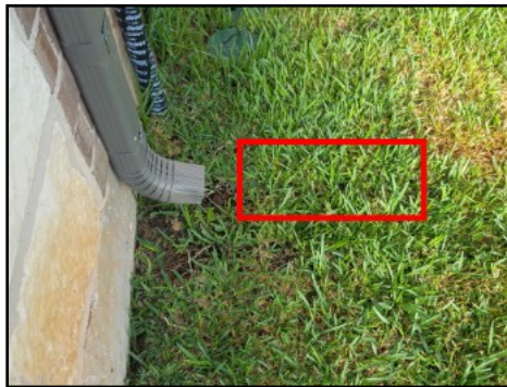
Missing splash block
