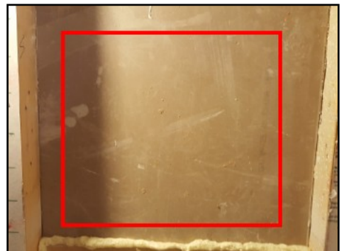
Insulation not present over scuttle door
