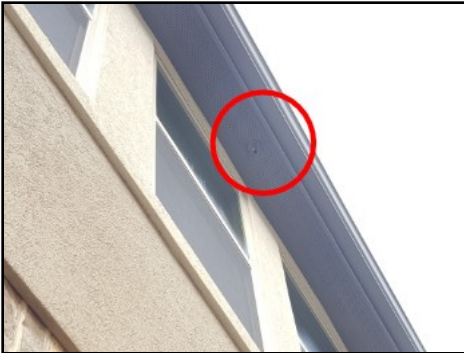
Secondary A/C drain line at rear right elevation
