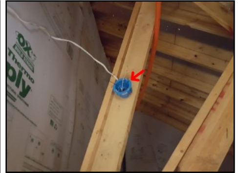
Light fixture/bulb missing
