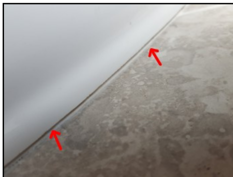
Master bathroom tub deck not sealed
