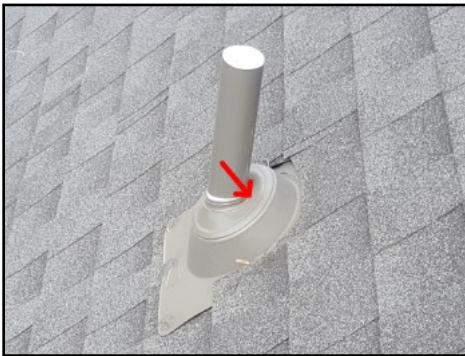
Buckled roof jack at upper rear left elevation
