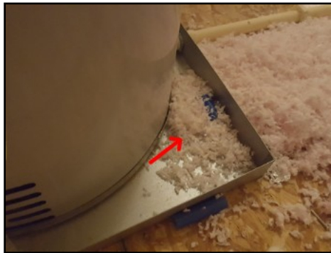
Debris in water heater drain pan
