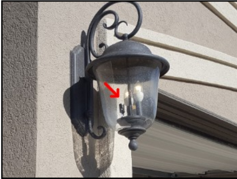
Light bulb missing at coach light
