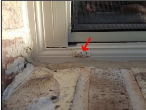
Blocked weep hole cover at rear left elevation
