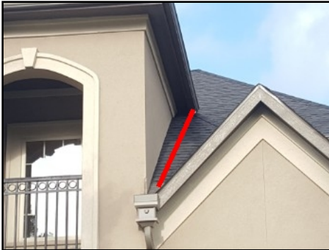
Gutter extension recommended
