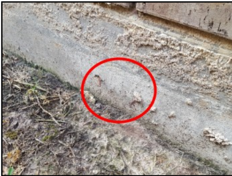
Remove nails from foundation wall
