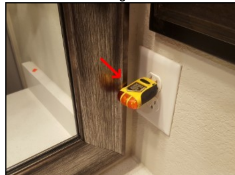
Receptacle blocked by mirror frame
