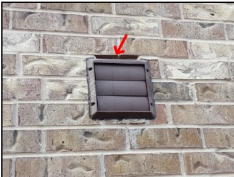
Seal all exterior penetrations
