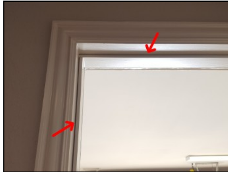
Missing weatherstripping at garage door
