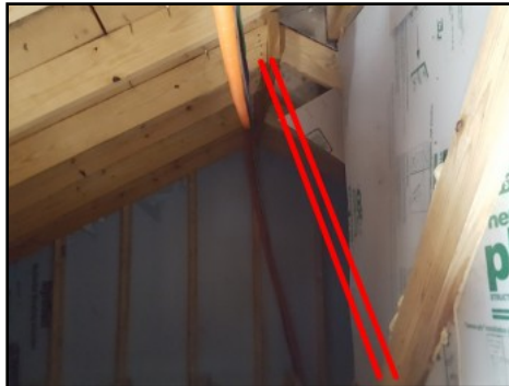
Ridge brace not present over 5' garage extension
