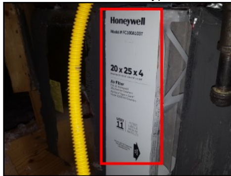
HVAC media filter type/size
