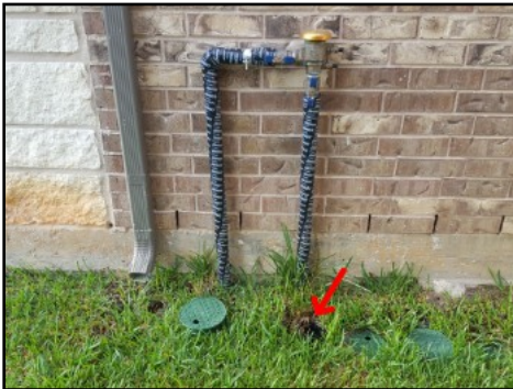
Main irrigation shut off valve
