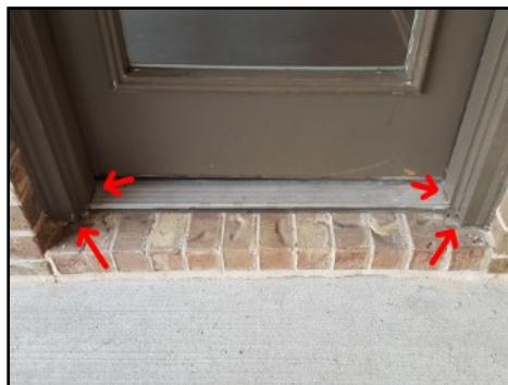
Seal door thresholds/jambs
