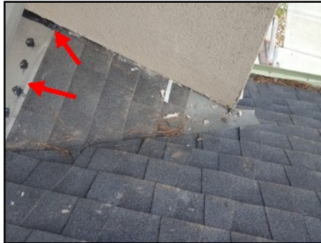
Fresh sealant at front elevation (over front garage)
