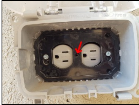
Front porch receptacle not secure
