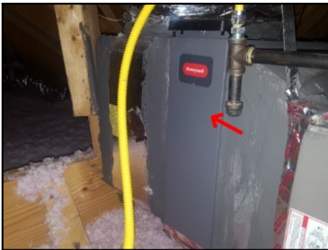
HVAC media filter location/hatch
