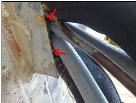
A/C refrigerant lines not sealed
