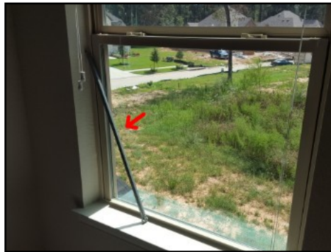
Sash track not secure in place
