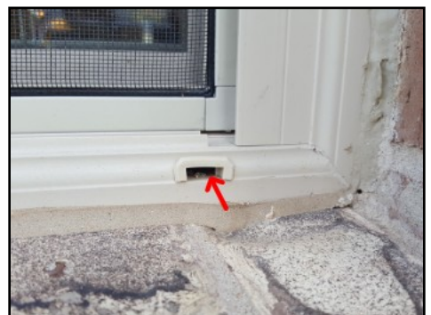
Damaged weep hole cover at rear elevation
