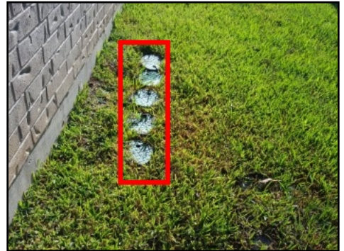
Possible leak at rear left valve
