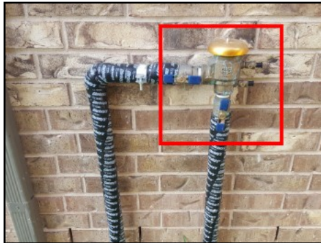
Homeowner service valves/anti-siphon device
