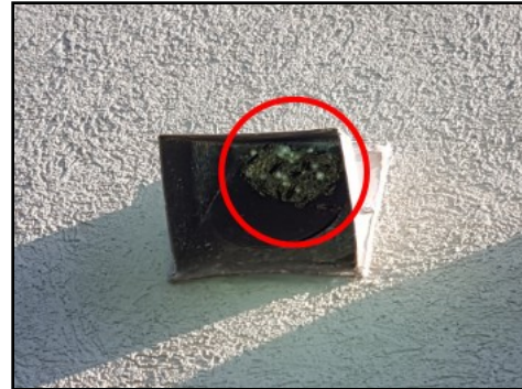
Damper blocked/Hornets nest present
