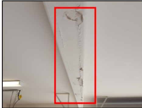
Moisture stains/damage present
