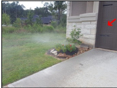
Sprinkler spraying structure
