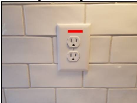
Missing sticker at GFCI receptacles
