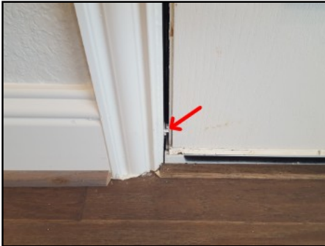
Gap at lower strike side
