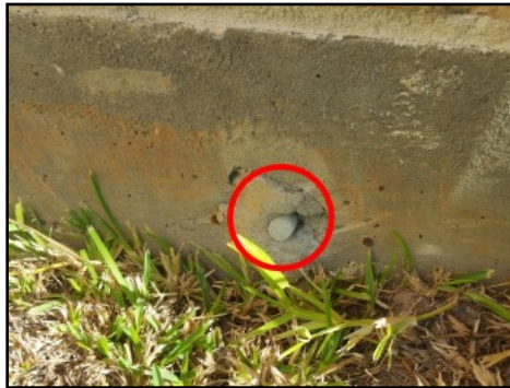
Exposed tension cable at left elevation
