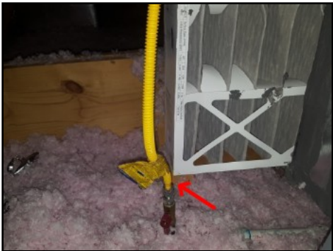
Gas line blocking HVAC media filter
