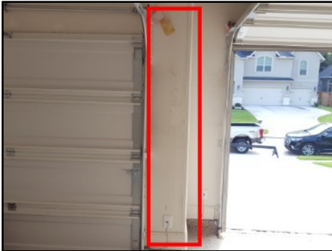
Moisture stains/damage present
