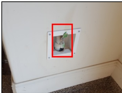
Main water shut off valve
