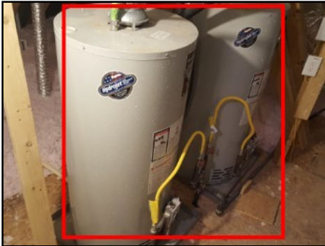
Water heaters located in lower attic space
