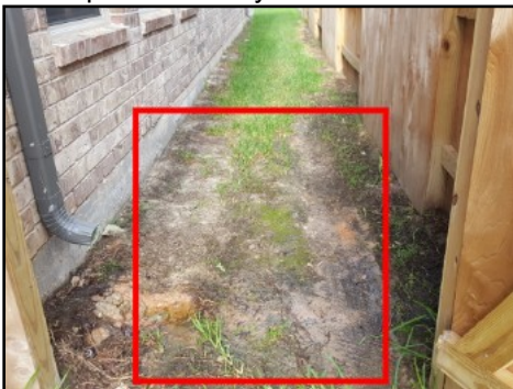
Evidence of excessive moisture
