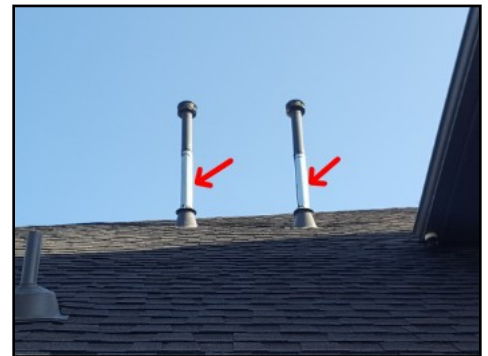
Vent pipes not painted
