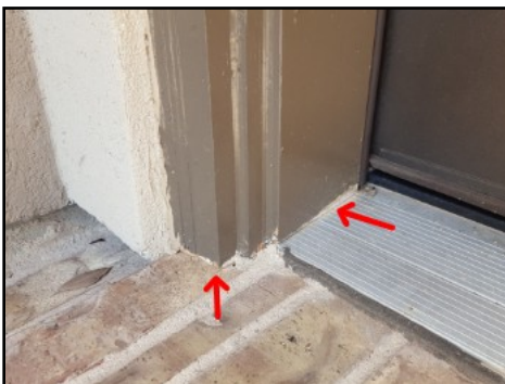
Seal door thresholds/jambs
