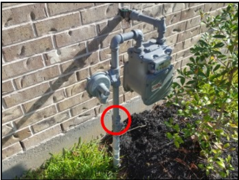
Gas meter and main shut off valve
