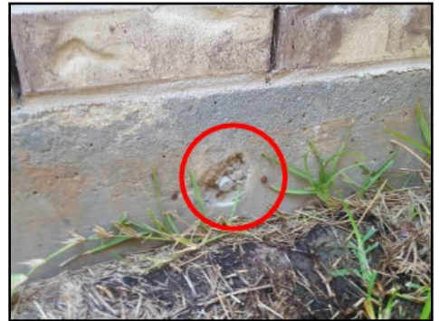
Exposed tension cable at rear left elevation
