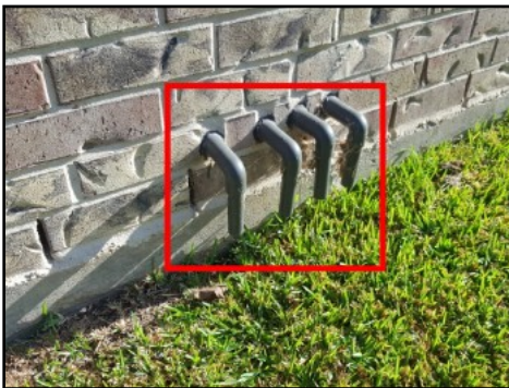
Drain line termination at rear left elevation
