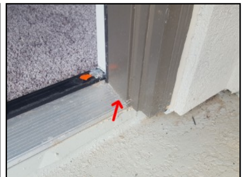
Seal door thresholds/jambs
