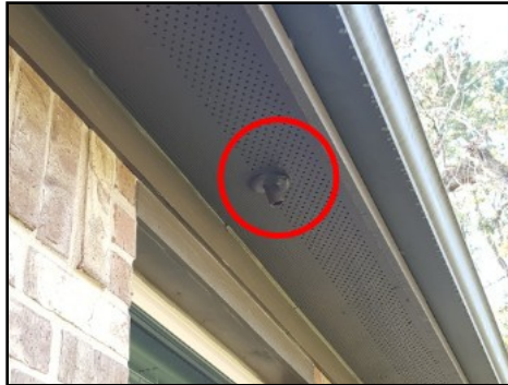
Secondary A/C drain line at rear elevation
