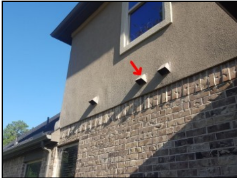
Dryer vent termination
