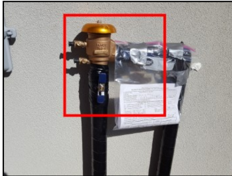
Homeowner service valves/anti-siphon device
