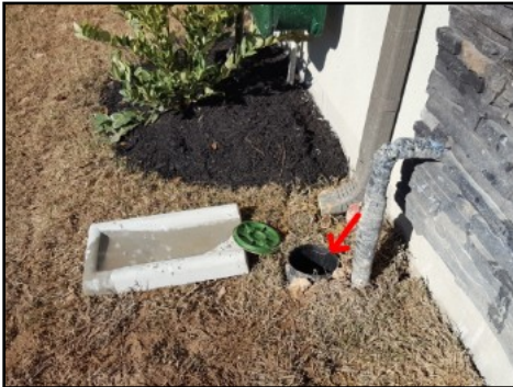
Main irrigation shut off valve
