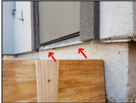
Seal rear elevation threshold
