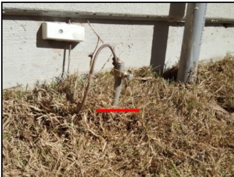
Ground rod not flush with grade
