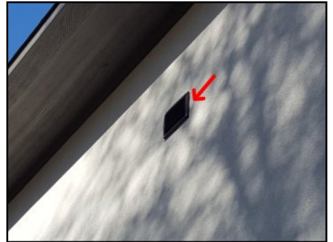
Seal all exterior penetrations
