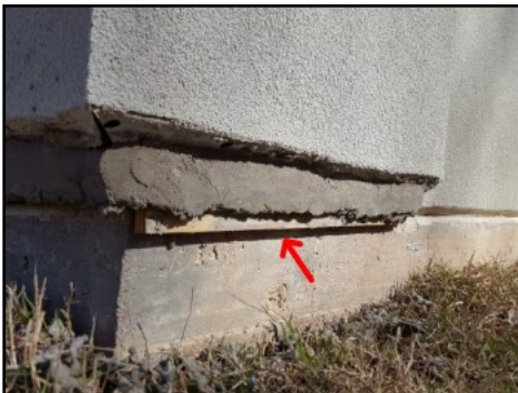
Remove wood at rear left column
