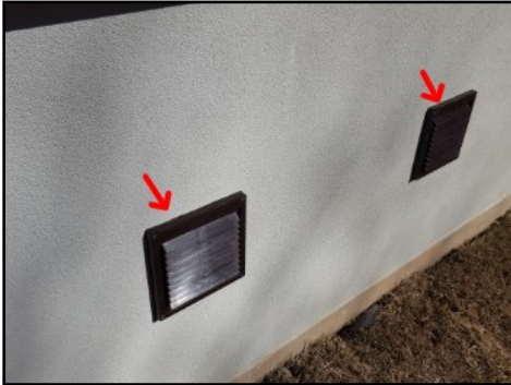
Seal all exterior penetrations
