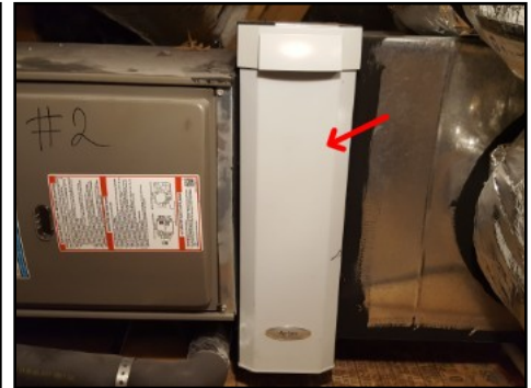
HVAC media filter location/hatch
