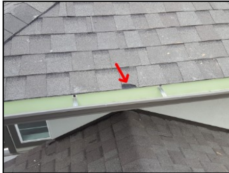
Damaged/torn shingle
