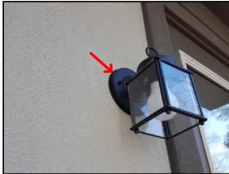
Seal all exterior penetrations
