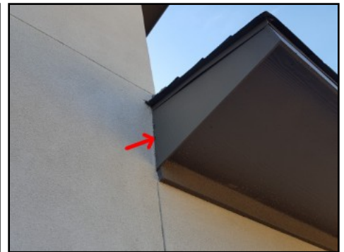
Seal material intersections
