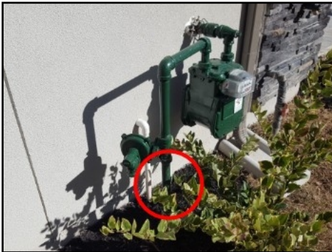
Gas meter and main shut off valve
