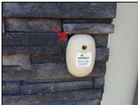
Seal all exterior penetrations
