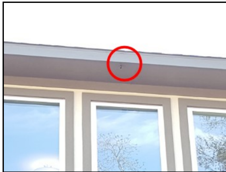
Secondary A/C drain line at rear elevation
