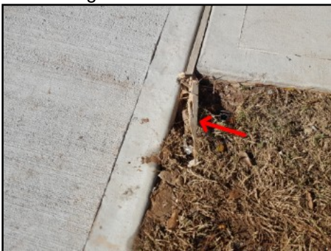
Flatwork expansion joint not removed
