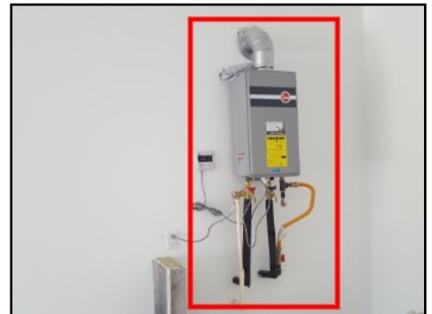
Tankless water heater located in garage
