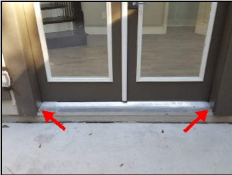
Keep door thresholds/jambs sealed
