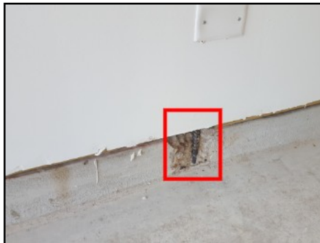
Foundation chipped at garage wall
