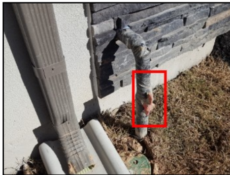
Main water shut off valve
