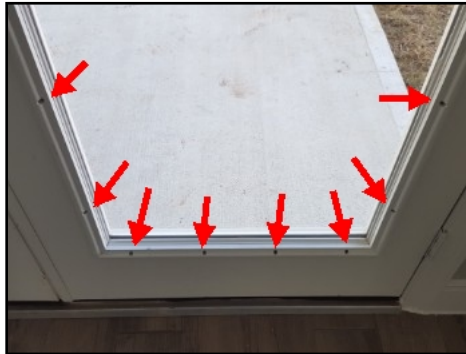
Missing screw caps/covers at back door
