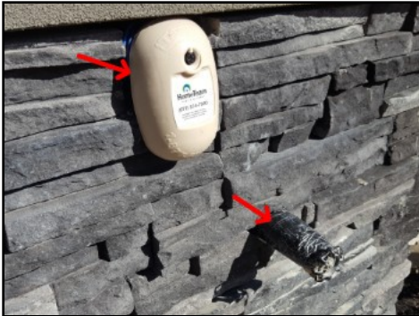
Seal all exterior penetrations
