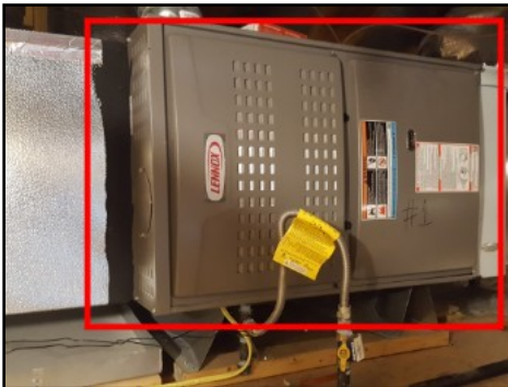
Furnace/Air handler located in upper attic space
