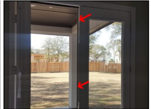
Missing weatherstripping at back door
