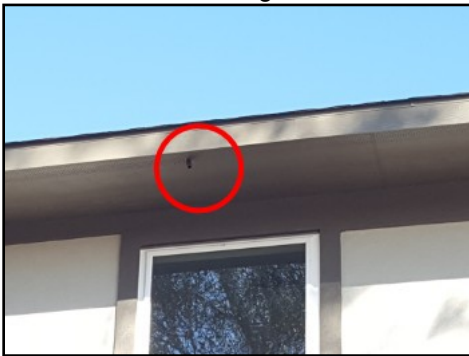
Humidifier drain line at rear left elevation
