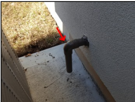
Drain line termination at rear left elevation
