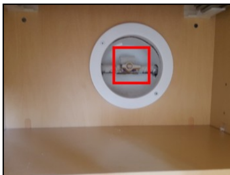
Gas line service valve within cabinet
