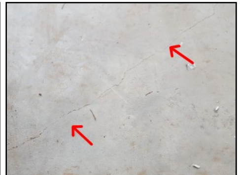
Hairline cracks in garage
