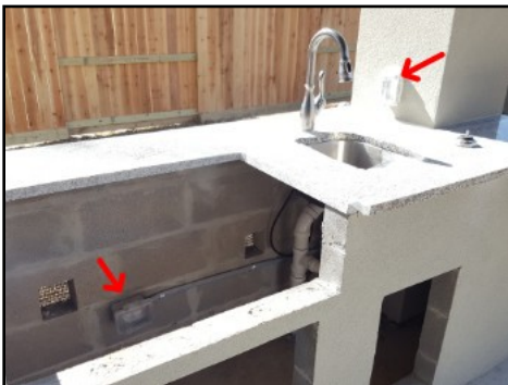
GFCI receptacles not functioning/resetting
