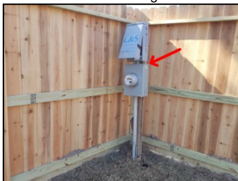
Remove temporary meter and pole
