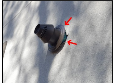
Repair stucco/Seal penetration
