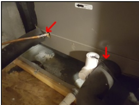
Seal refrigerant/drain lines at evaporator coil cabinet
