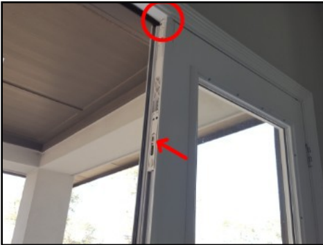
Flush bolt inoperable at back door
