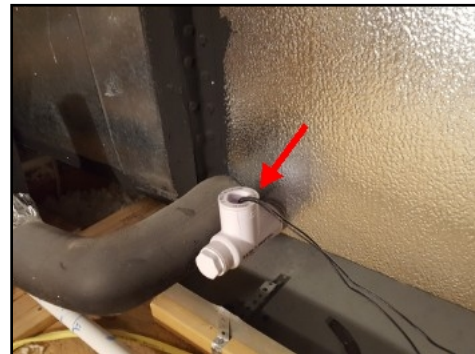
Seal drain lines at evaporator coil cabinet
