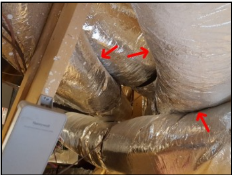
HVAC duct work in contact with one another
