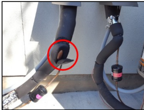
Damaged/torn refrigerant line insulation
