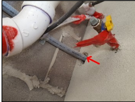
Seal all exterior penetrations
