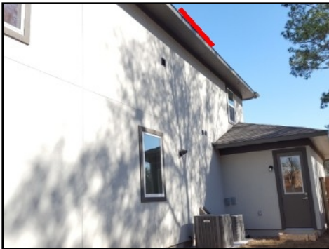
Recommend splash guard over condensing units
