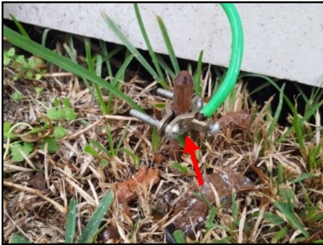
Incorrect ground clamp
