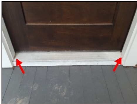
Seal door thresholds/jambs
