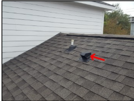
Dryer vent termination
