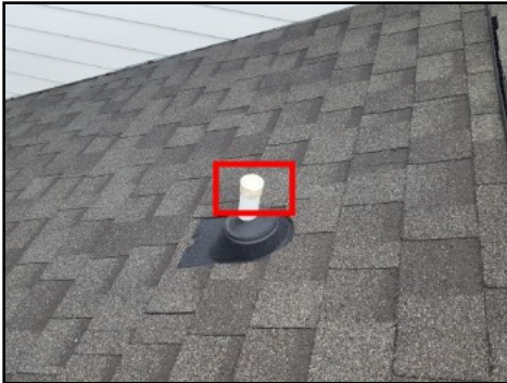
Stack vent capped/covered
