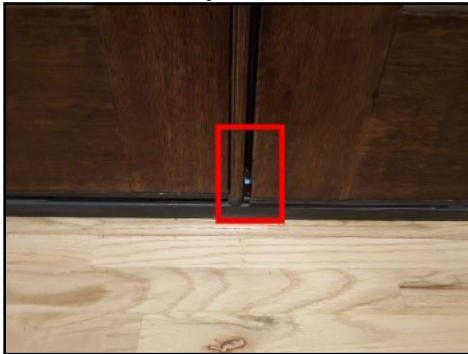
Gap at lower strike side
