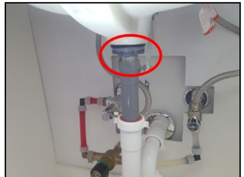
Leak present at master bathroom vanity drain
