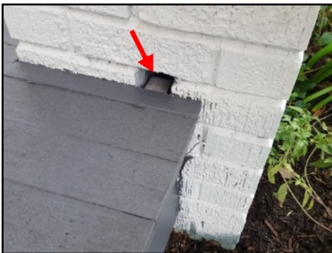
Seal material intersections
