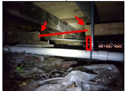
Floor joist altered/not supported
