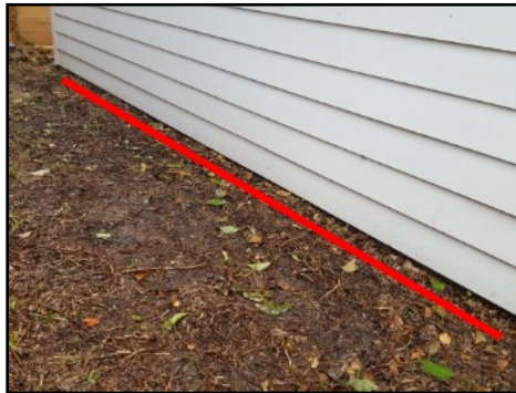
High grading at detached garage
