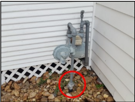
Gas meter and main shut off valve
