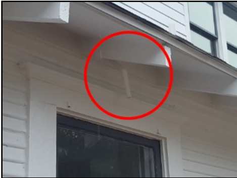
Secondary A/C drain line at rear right elevation
