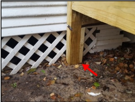
Post material in contact with grade/soil
