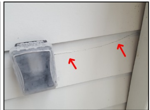
Damaged/cracked siding material at rear elevation
