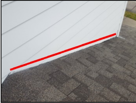
Siding in contact with shingles
