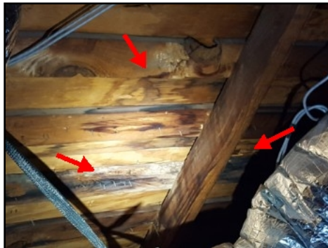
Moisture stains present at attic deck/lumber
