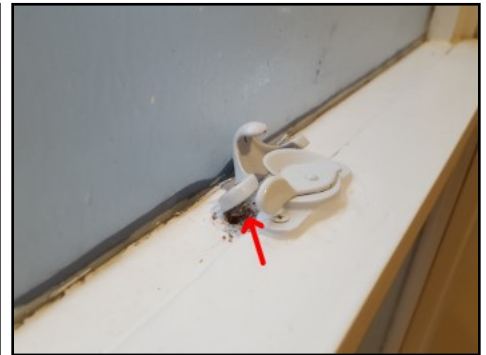
Latch housing not secure in place
