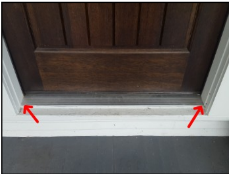
Seal door thresholds/jambs
