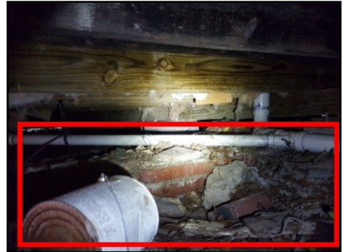
Debris/voids present within crawlspace
