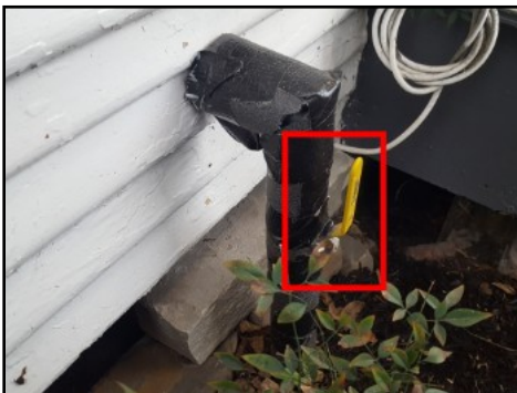
Main water shut off valve
