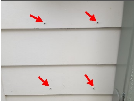
Seal holes in siding at rear left elevation
