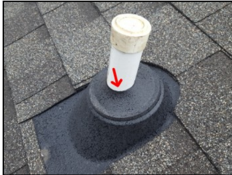
Stack vent/roof jack not sealed
