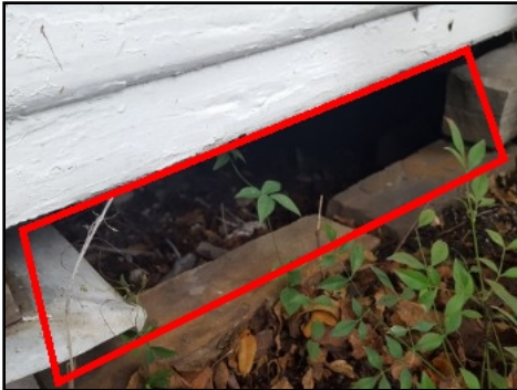
Skirt/cover not present at crawlspace
