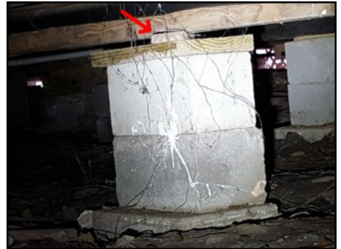
Inadequate beam support within crawlspace
