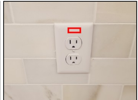
Missing sticker at GFCI receptacles
