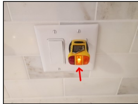
"Open ground" at GFCI receptacle
