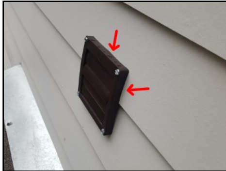
Seal all exterior penetrations
