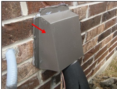
Example of rain hood flashing
