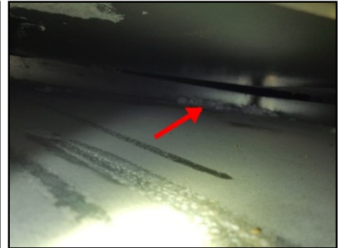
Debris in secondary A/C drain pan
