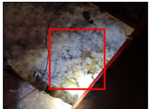
Compressed/missing insulation
