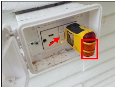
GFCI inoperable/Not resetting
