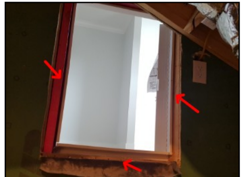
Attic door jamb not foam sealed
