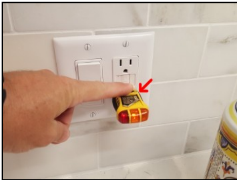
GFCI receptacle not tripping
