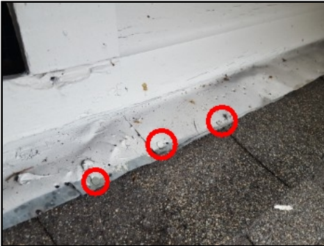
Exposed nails at roof covering
