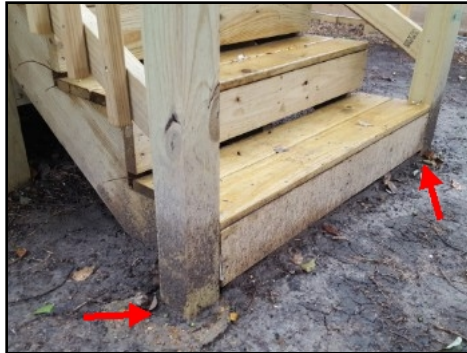
Post material in contact with grade/soil
