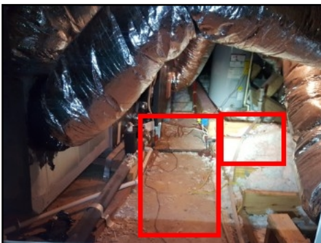
Improper walkway/landing in attic space
