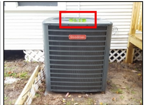
Condensing unit not level
