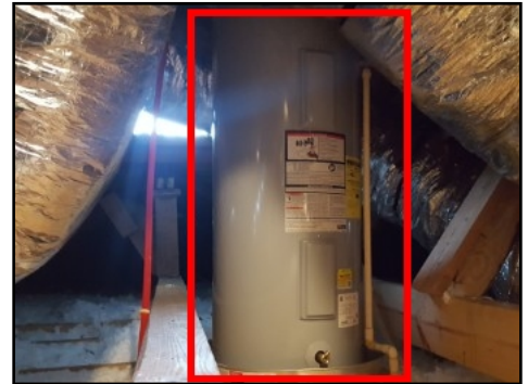
Water heater located within the lower attic space
