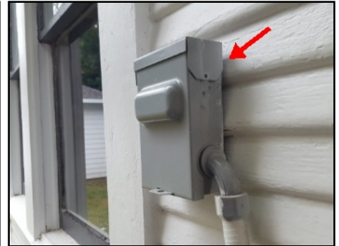
Seal all exterior penetrations
