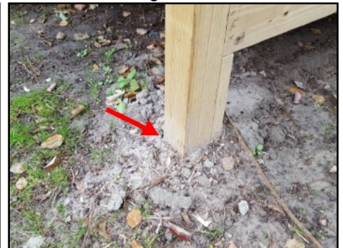
Post in contact with grade/soil
