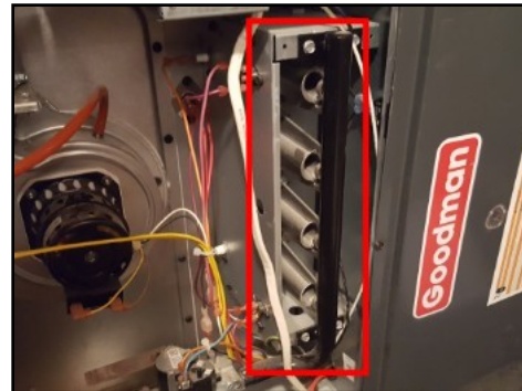
Furnace burner ports
