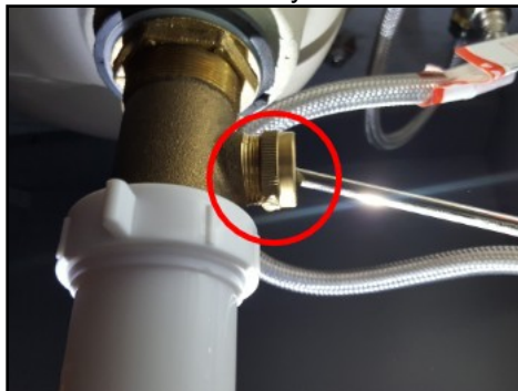
Leak at lower bathroom vanity drain stop
