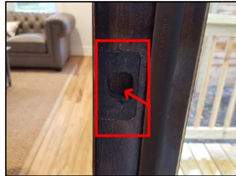
Missing strike plate/bore deadbolt hole
