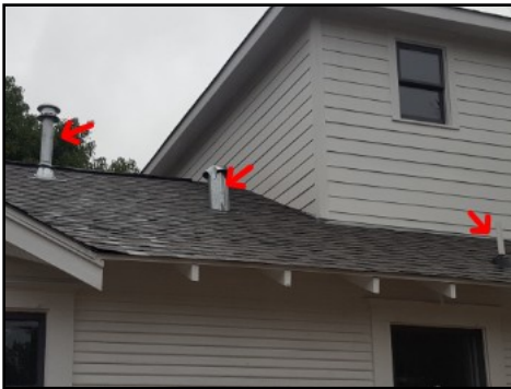
Vents/roof jacks not painted at right elevation
