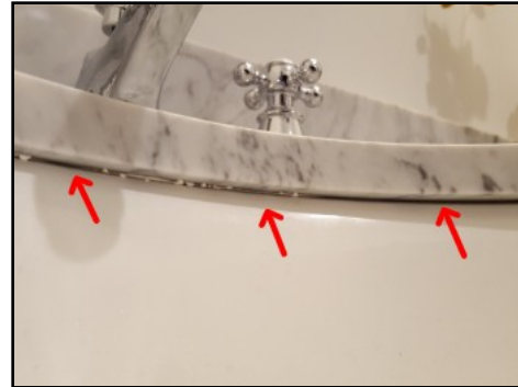
Bathroom vanities not sealed at counter top
