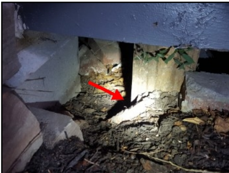
Post material in contact with grade
