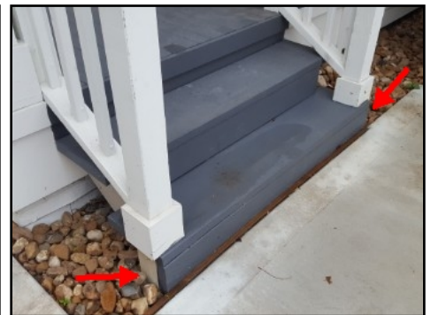
Rear porch material in contact with grade
