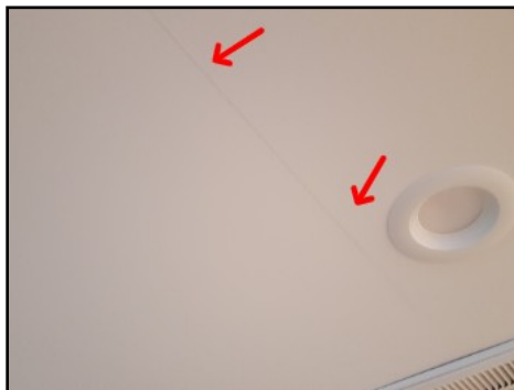
Settling crack at living room ceiling
