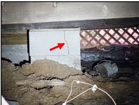
Pier material cracked within crawlspace
