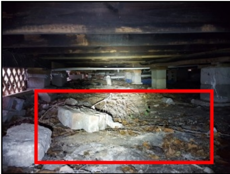
Debris/voids present within crawlspace
