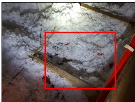
Compressed/missing insulation
