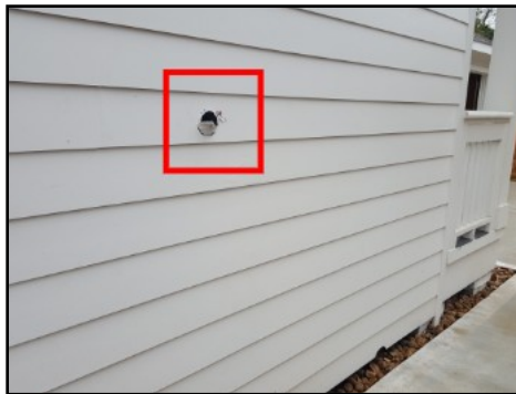
Vent cover not present/Seal exterior penetrations
