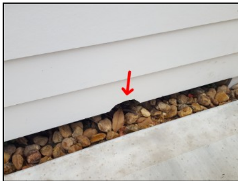
Damaged siding material at rear right elevation
