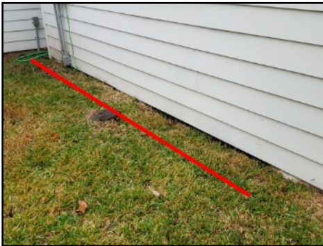
High grading at rear elevation
