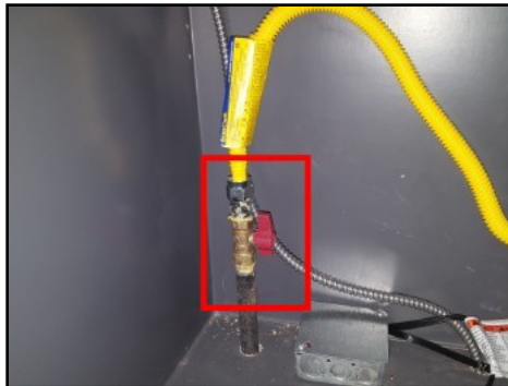
Gas line service valve is beneath unit
