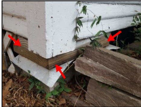
Exposed lumber at front left corner
