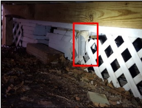
Drain line termination at rear left elevation
