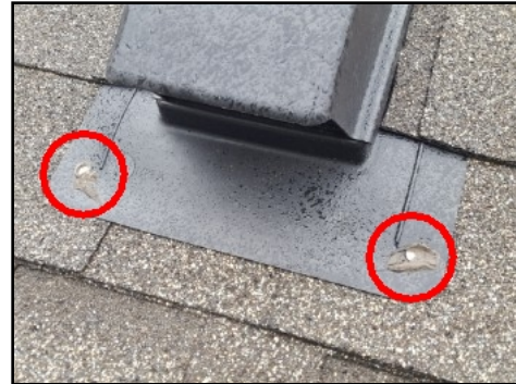
Exposed nails at roof covering
